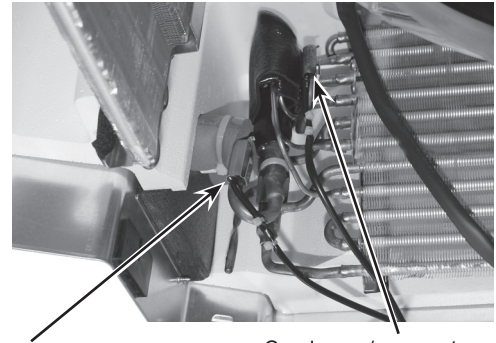
Pipe temperature/liquid thermistor (TH2)
