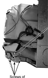
Screws of the vane motor unit cover
