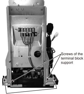
Screws of the earth wires and the terminal block support
