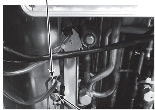
High pressure switch (63H)
